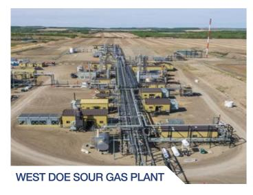
FEED and Detail Design for a sour gas plant with three process trains totaling 100 TJ with process gas conditions of 2.6% H2S and 3.0% CO2 from the Montney.
