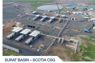
FEED, Detail Design and installation for brownfield plant expansion from 30 TJ to 90 TJ utilizing existing Standard Design package for gas processing plant design. Project includes inlet gas manifold, main compression, booster compression, TEG dehydration, fuel gas skid, sales gas metering, utilities, as well as water treatment.
