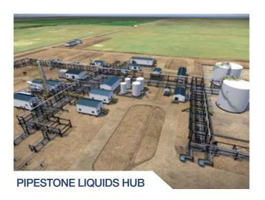
FEED, Detail Design and Installation of 30,000 bbl/d Liquids Terminal & Pumping Station, including 22,000 bpd pf sour condensate and 8,000 bbl/d of produced water. Major equipment includes inlet separation, condensation stabilization, mercaptan removal, compression, pump packages, condensate storage (15,000 bbl), water storage (10,000 bbl), power, utilities.
