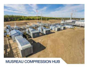
FEED, Detail Design and installation of 50 TJ single train gas plant. Facility includes inlet separation, condensate stabilization, inlet compression, sales compression, refrigeration, de-ethanizer, vapour recovery unit, power generation, recycle system, storage for produced water, condensate and NGL.
