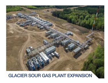
Equinox executed the FEED and Detail Design for the brownfield sour gas plant expansion to 250 TJ capacity. Newly installed facilities include refrigeration, condensate stabilization, compression, vapour recovery unit, power generation as well as an upgraded amine sweetening plant.
