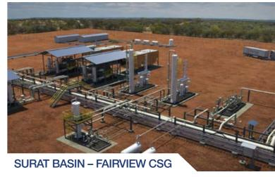
Development of 'Standard Design' 60 TJ Central Processing Facility (including inlet header, slug catcher, compression, dehydration, coalescer and metering).
