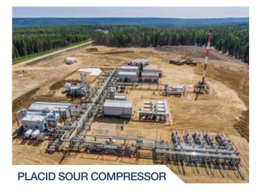
FEED, Detail Design and installation for 60 TJ sour processing facility with 16,000 bpd of liquids. Fast tracked (9 month) schedule including engineering through to commissioning and start-up. Equipment includes inlet module for multiphase gathering lines, inlet separation, compression, dehydration, emulsion pump package, instrument air, fuel gas, MCC building, power generation, LP and HP flare, office / control building.
