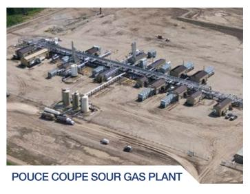
FEED, Detail Design and installation of 60 TJ dual train, sour gas plant. Processing trains (2 x 30 TJ) include inlet separation, inlet/sales compression, amine sweetening, refrigeration, liquid fractionation and stabilization, acid gas compression, vapour recovery, recycle system, storage for produced water, condensate and NGL.
